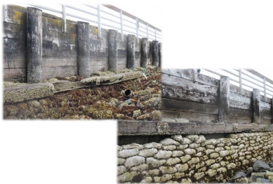
Figure 2-13. Old North & West Timber Pile Bulkhead
