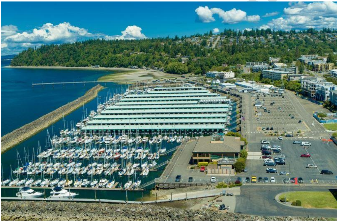
Figure 1. City of Des Moines Marina
