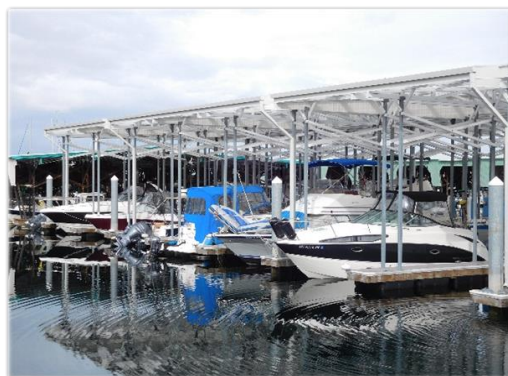
Figure 4-2. Covered Moorage on J-Dock
