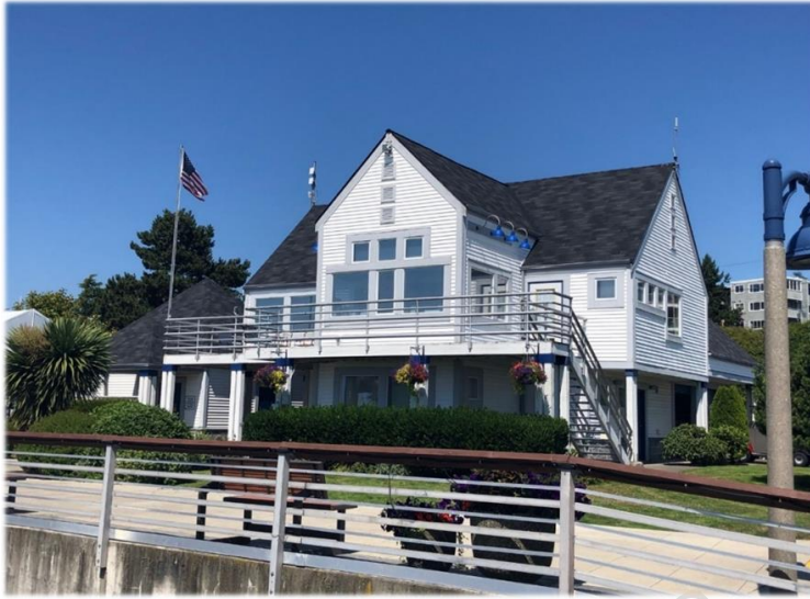
Figure 5-1. Marina Office Building July 2021
