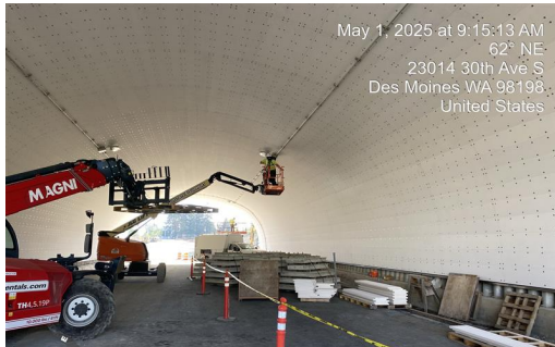
Crews install fireproofing panels and a waterline under the Veterans Drive tunnel.
