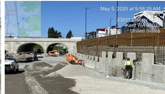
Crews placing concrete barrier for the new eastbound SR 516 to northbound I-5 ramp.
