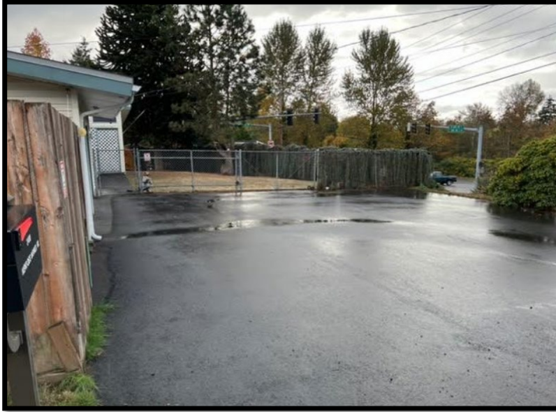
Facing South Towards the Proposed Acquisition Area.
