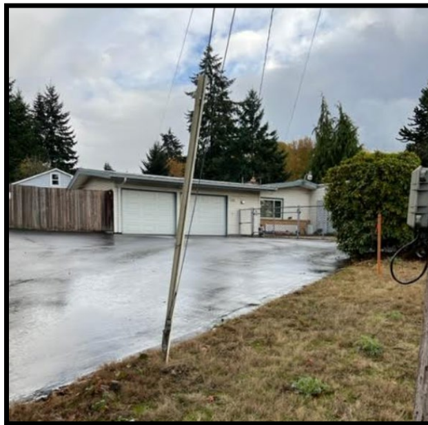
Facing SE Towards the Subject Residence.
