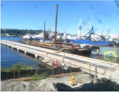
Ballard Tunnel Pier Replacement - $9,371,000
