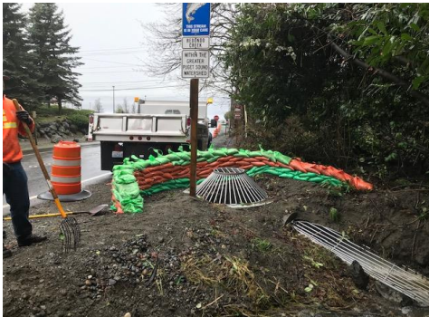
Sand bag installation after January 2021 overflow event
