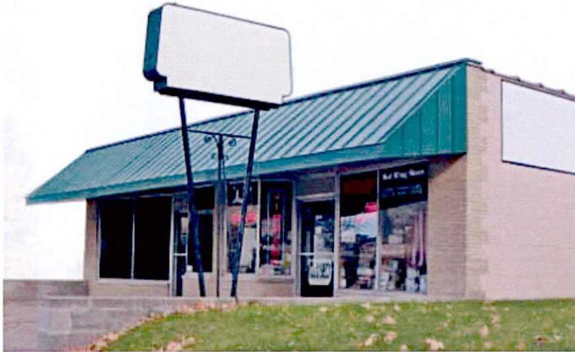
Before: This large metal awning overwhelms the small building.
