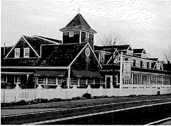
The varied rooflines of this Harwich building add visual interest.
