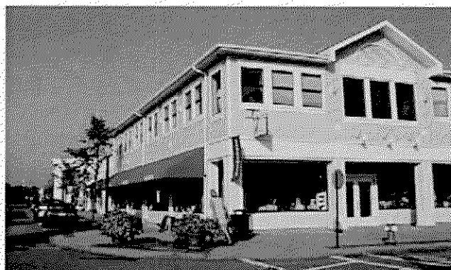
An example of a contemporary two-story commercial building in Mashpee that provides a mix of retail and office space within a two-story structure
