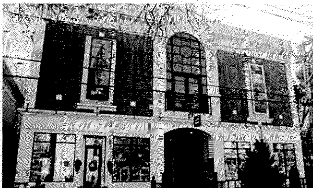
This reconstructed two-story commercial building in Provincetown incorporates large upper-level windows to allow light into the building.
