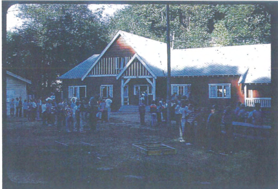
West side of Dining Hall, painted red with white trim. (undated)
