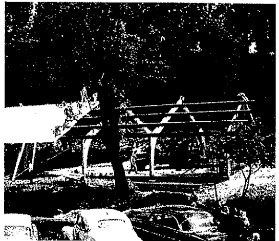
ca. 1956 photograph of the Auditorium during construction. Source: Steve Gilchrist.
