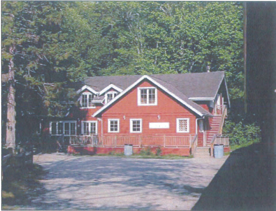
Sun Home Lodge from the west, showing the addition (cross gable at center), likely from a 1981 remodel.
