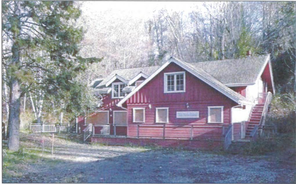
West facade of Sun Home looking northeast. Note windows are boarded up, and pickets are missing from deck railings.
