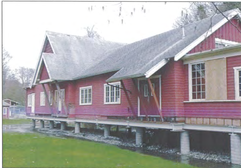
West side of the Dining Hall looking north.
