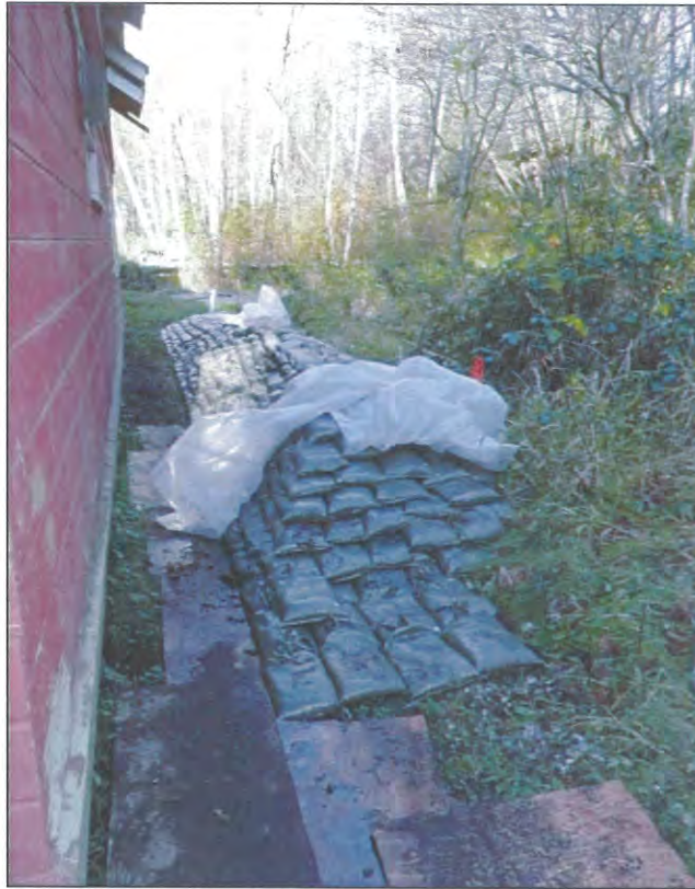
East side of Sun Home Lodge looking north, with temporary sandbag berm installed close to the building.
