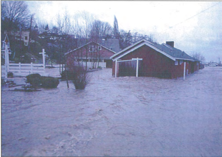
Washrooms at right with Picnic Shelter beyond (far right) and Dining Hall at center in the distance. The 2007 flood was clearly not the first! (undated)
