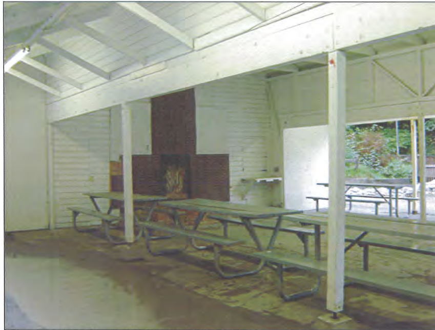
Interior of the Picnic Shelter, looking northeast.
