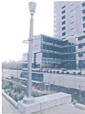
Pedestrian area lighting
