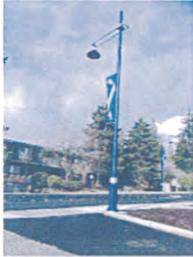
Parking lot lighting
