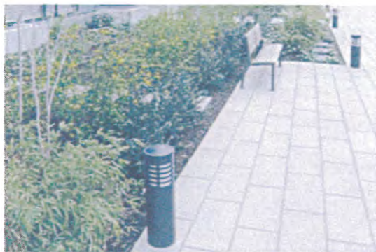
Use of bollards as pedestrian pathway lighting
