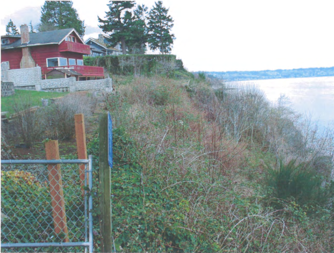
Adjacent Property- Bluff Looking South
