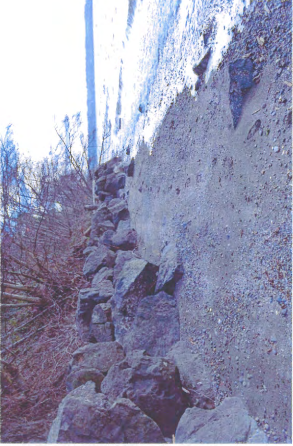
Existing Bulkhead Looking South
