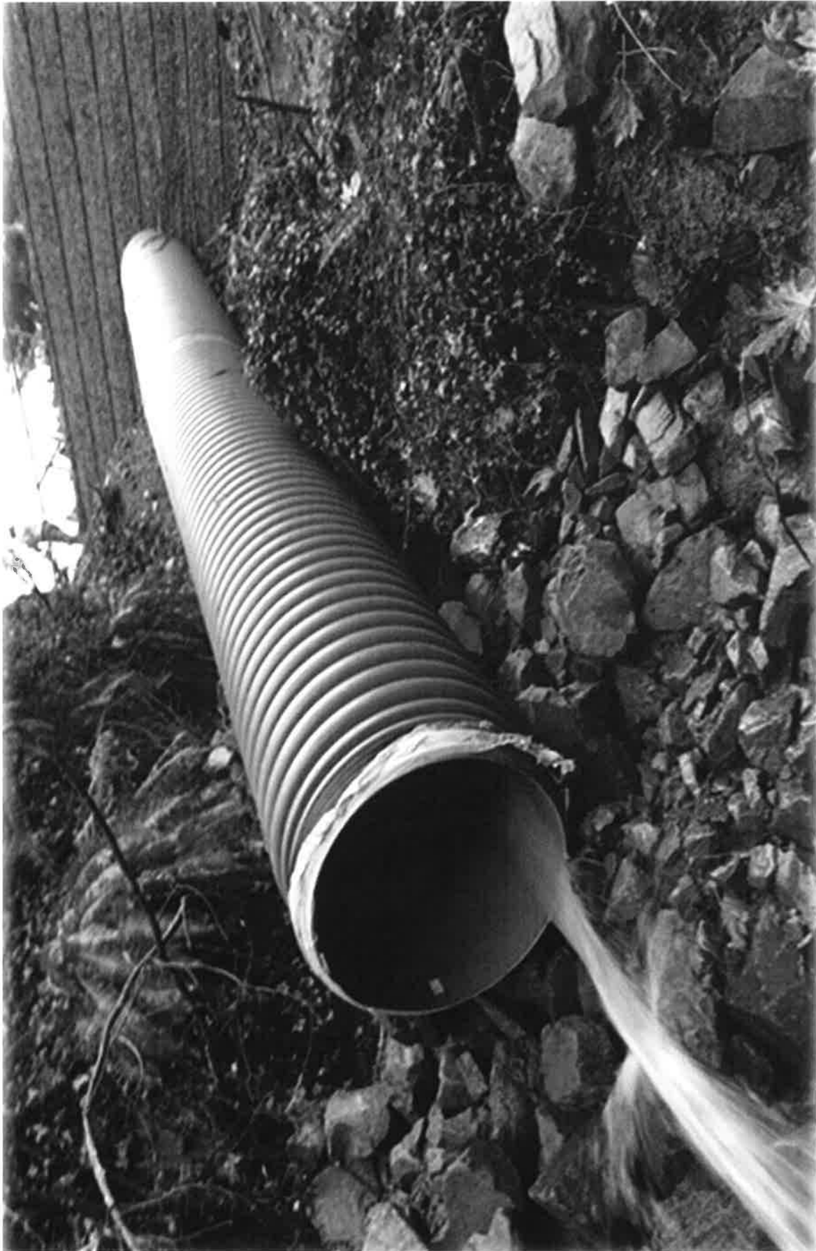
S. 251st Street Storm Outfall
