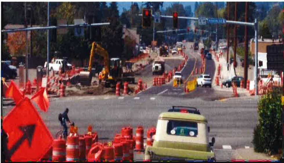
S. 216th Street – looking west (8-16-2016)
