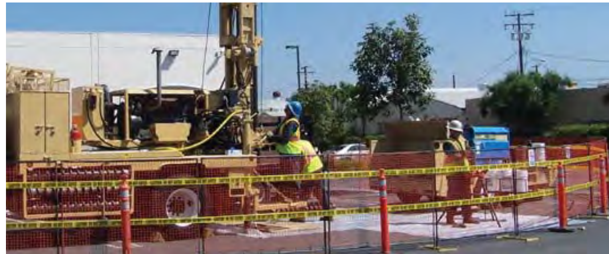
Geotechnical borings
