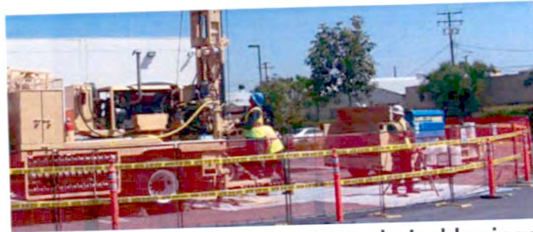
Geotechnical borings
