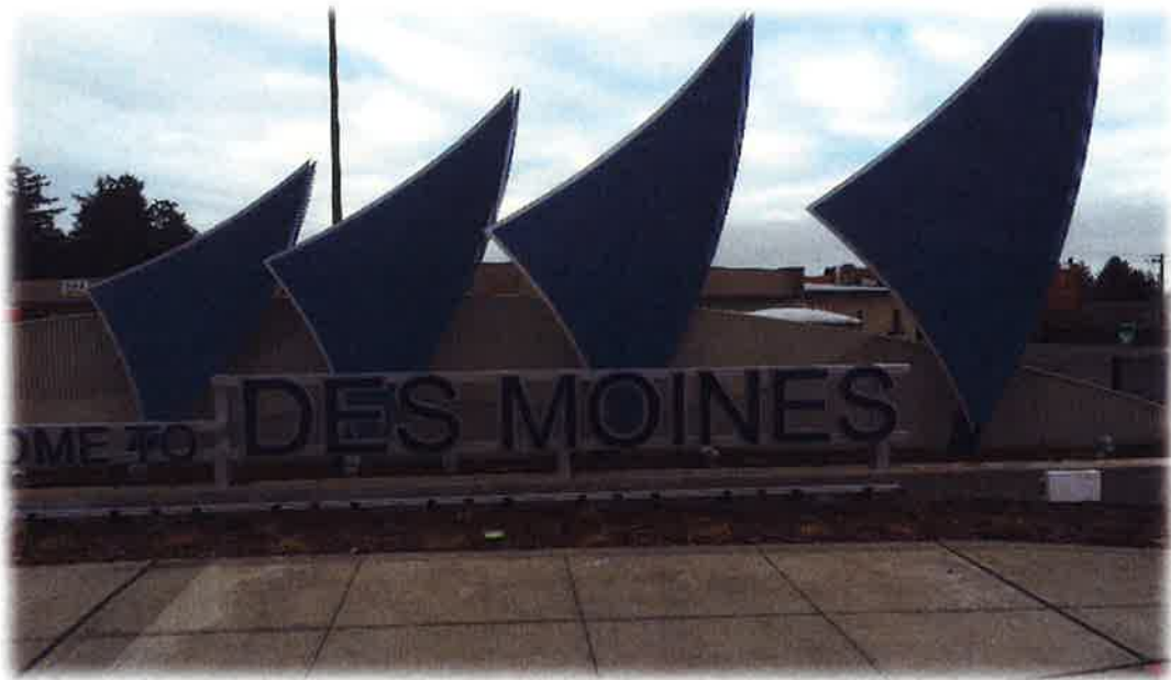
New Gateway Decorative Wall (1-24-2017)
