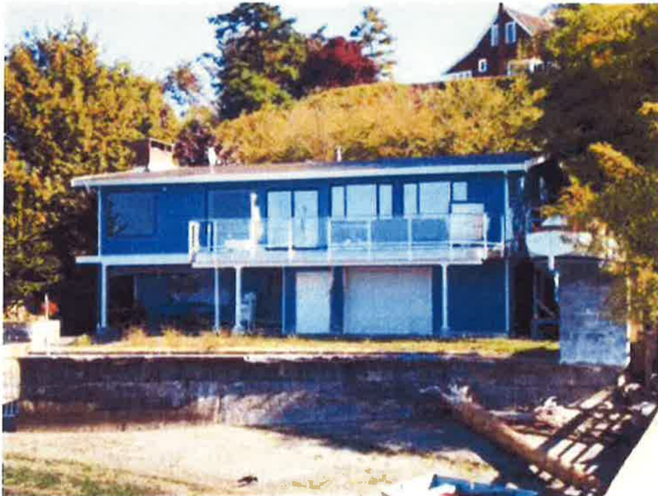
Figure 3: view of west side of residence.
