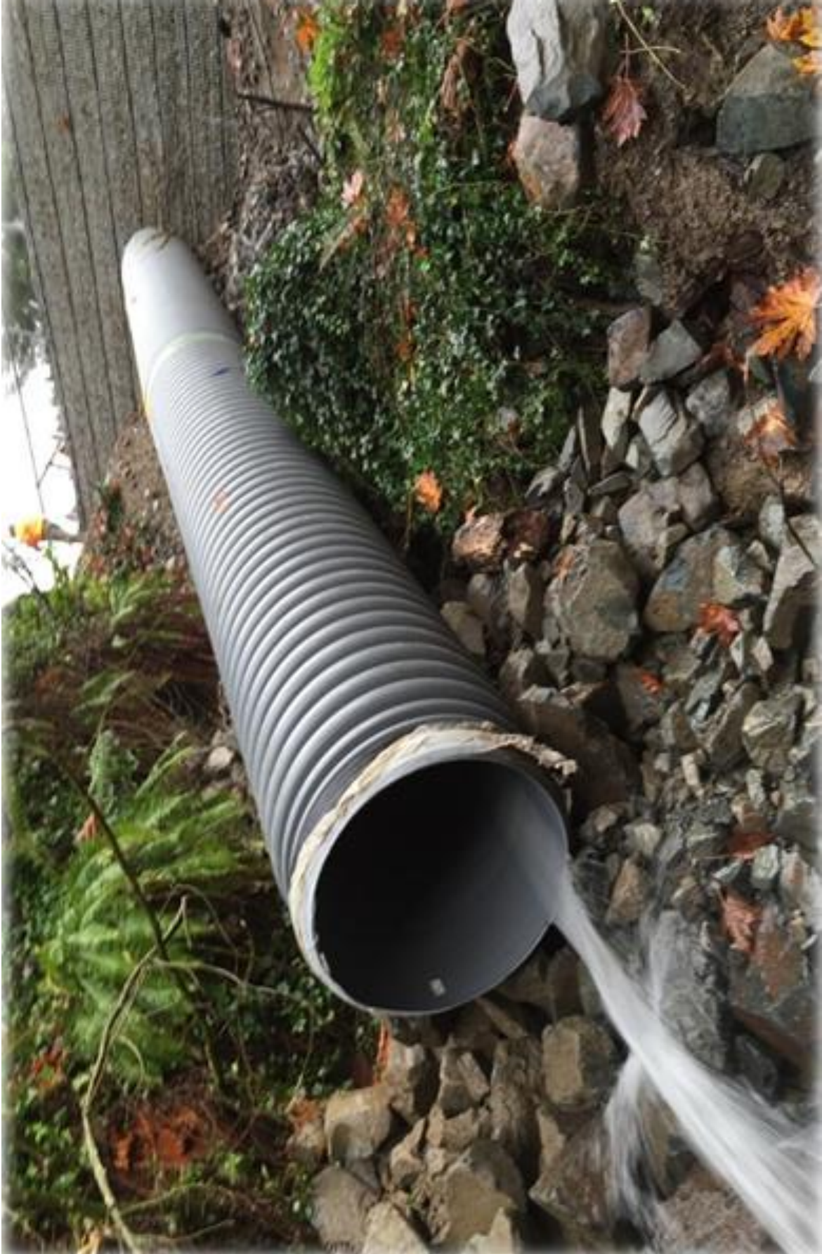
S. 251st Street Storm Outfall
