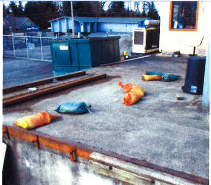
(AFTER) Photo 14-A: POLLUTION GENERATING MATERIALS HAVE BEEN RELOCATED UNDER COVER OR DISPOSED OF PROPERLY. AREA HAS BEEN SWEEPED.
