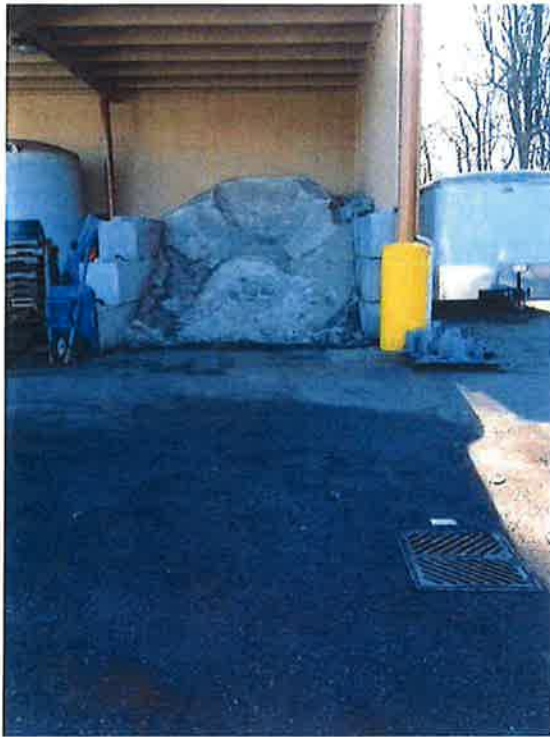
05 DESCRIPTION: COVERED SALT PILE IN CLOSE PROXIMITY TO CATCH BASIN
