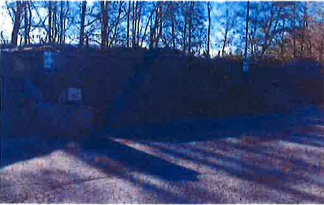
(BEFORE) Photo 11: UNCOVERED MATERIAL STORAGE BAYS.
