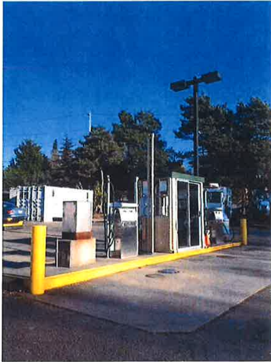
13 DESCRIPTION: FUELING ISLAND
