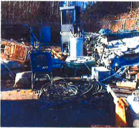
(BEFORE) Photo 01: NW CORNER MATERIAL STORAGE. POLLUTION GENERATING MATERIAL EXPOSED TO RAINFALL.
