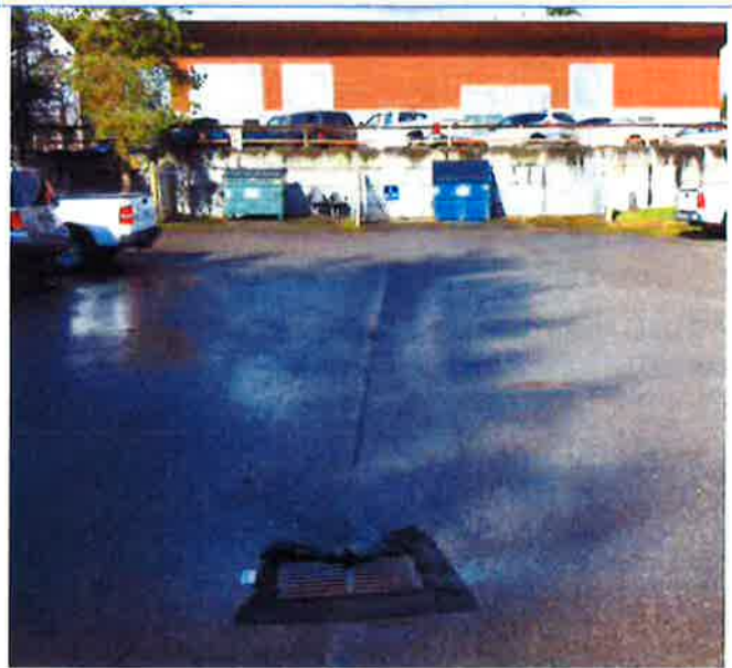
(AFTER) Photo 06-A: GARBAGE AND RECYCLING DUMPSTERS HAVE BEEN CLOSED. STAINING FROM VEHICLE FLUIDS HAVE BEEN MANAGED AND FILTER FABRIC SOCKS HAVE BEEN INSTALLED.
