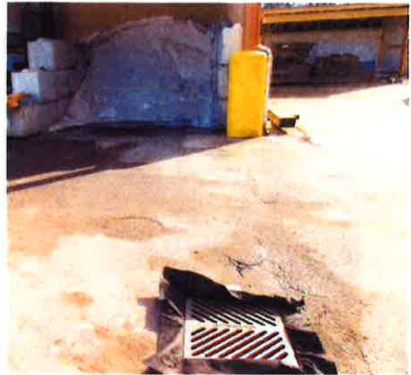
(AFTER) Photo 05-A: AREA PAVEMENT SWEEPED. SALT BAY IS STILL WAITING FOR A NEW BERM. PHOTO SHOWS A FOURTH NEWLY CONSTRUCTED COVERED AREA.
