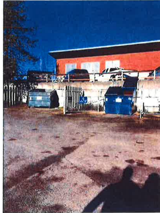
06 DESCRIPTION: GARBAGE AND RECYCLING DUMPSTERS LEFT UNCOVERED. SOME STAINING FROM VEHICLE FLUIDS VISIBLE ON PAVEMENT.
