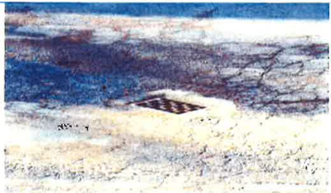
(AFTER) Photo 09-A: AREA HAS BEEN SWEEPED. THE ASPHALT BAY STILL NEEDS TO HAVE A BERM INSTALLED.
