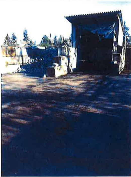
09 DESCRIPTION: TRACKOUT FROM ASPHALT STORAGE BAY.
