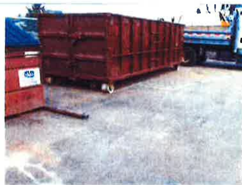
(AFTER) Photo 02-A: POLLUTION GENERATING MATERIAL HAS BEEN RELOCATED OR DISPOSED OF PROPERLY. AREA HAS BEEN SWEEPED.
