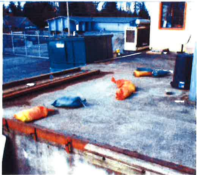
(AFTER) Photo 14-A: POLLUTION GENERATING MATERIALS HAVE BEEN RELOCATED UNDER COVER OR DISPOSED OF PROPERLY. AREA HAS BEEN SWEEPED.
