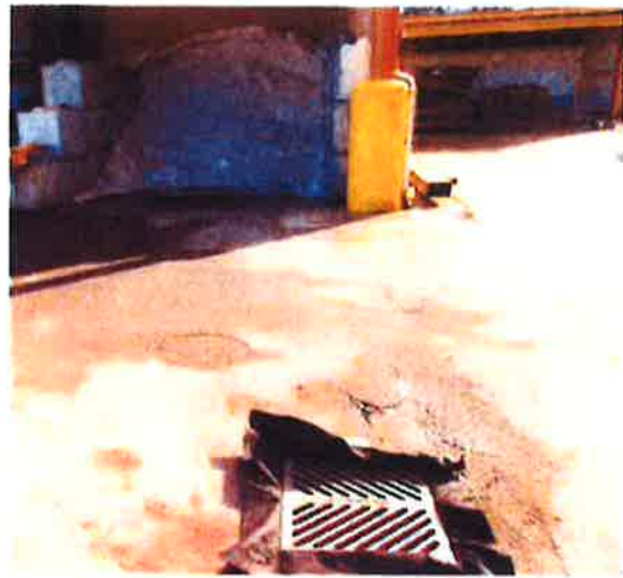
(AFTER) Photo 05-A: AREA PAVEMENT SWEEPED. SALT BAY IS STILL WAITING FOR A NEW BERM. PHOTO SHOWS A FOURTH NEWLY CONSTRUCTED COVERED AREA.
