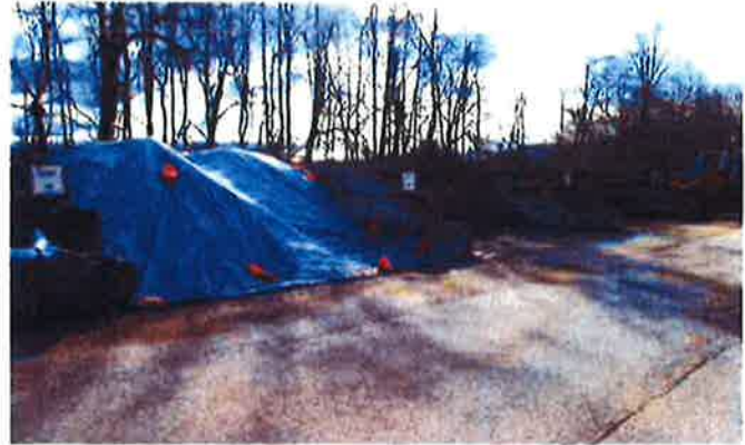
(AFTER) Photo 11-A: PHOTO SHOWS ONE OF THREE MATERIAL BAYS COVERED. MATERIAL BAYS STILL NEED INTERIUM COVERS INSTALLED AND BERMS INSTALLED. AREA HAS BEEN SWEEPED.
