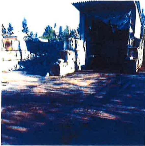
(BEFORE) Photo 09: TRACK OUT FROM ASPHALT STORAGE BAY.
