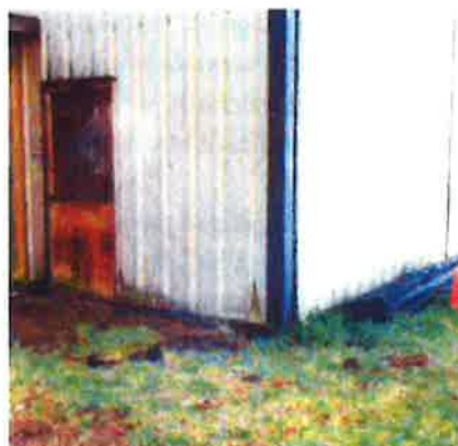
(AFTER) Photo 02-A: BARREL HAS BEEN DISPOSED ON PROPERLY AND REMOVED FROM THE SITE
