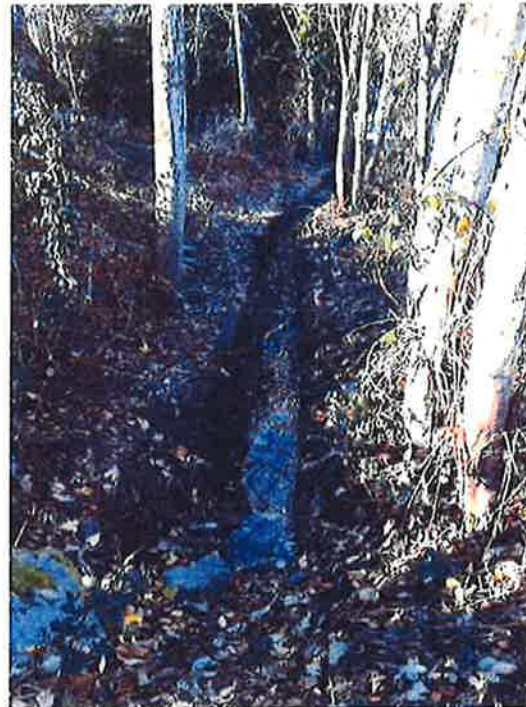
16 DESCRIPTION: RECENTLY EXCAVATED UNSTABILIZED DITCHLINE FROM WESTERN STORMWATER CONVEYANCE AND DETENTION PIPE TERMINUS TO STREET DITCHLINE. TERMINUS OF ON-SITE STORMWATER SYSTEM AT BOTTOM OF PHOTO.
