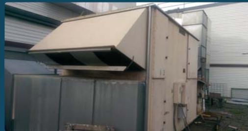
Air Handler Replacement
