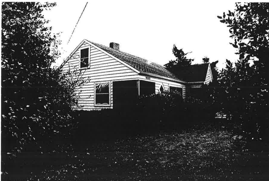
Front view of 24728 16th Avenue South viewed to the southwest from the northerly driveway.
