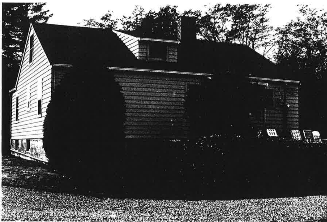
Rear view of 24728 16th Avenue South.
