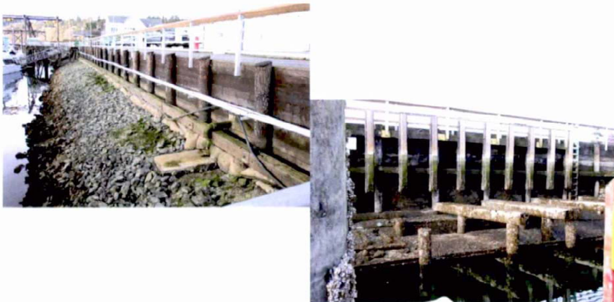
Figure 2-2. Timber Pile Bulkhead
