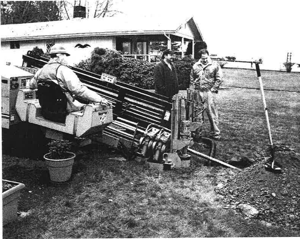
Exhibit #1: Directional Bore Machine
