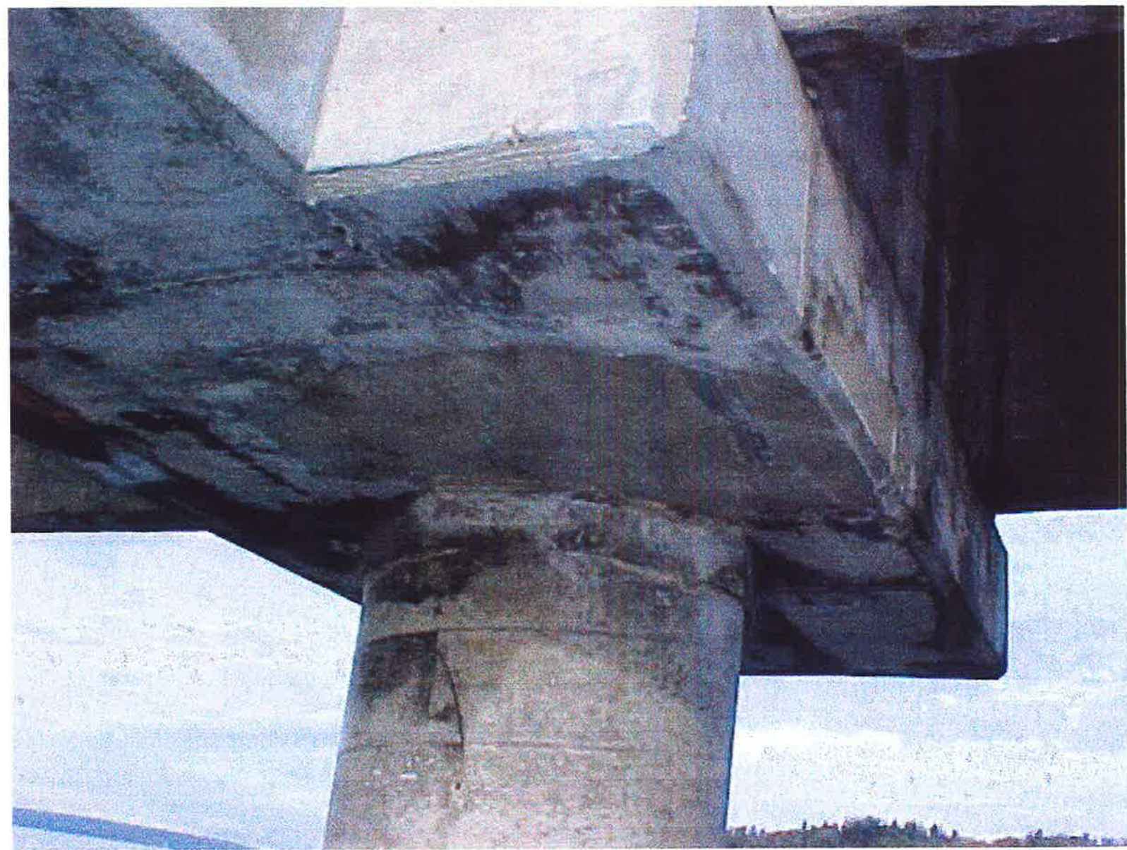
Repair to Bent #6 complete
