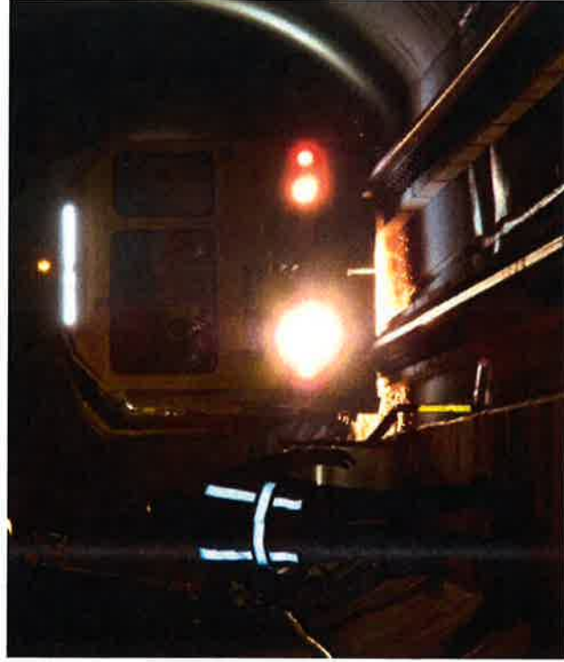
Rail surface grinding
