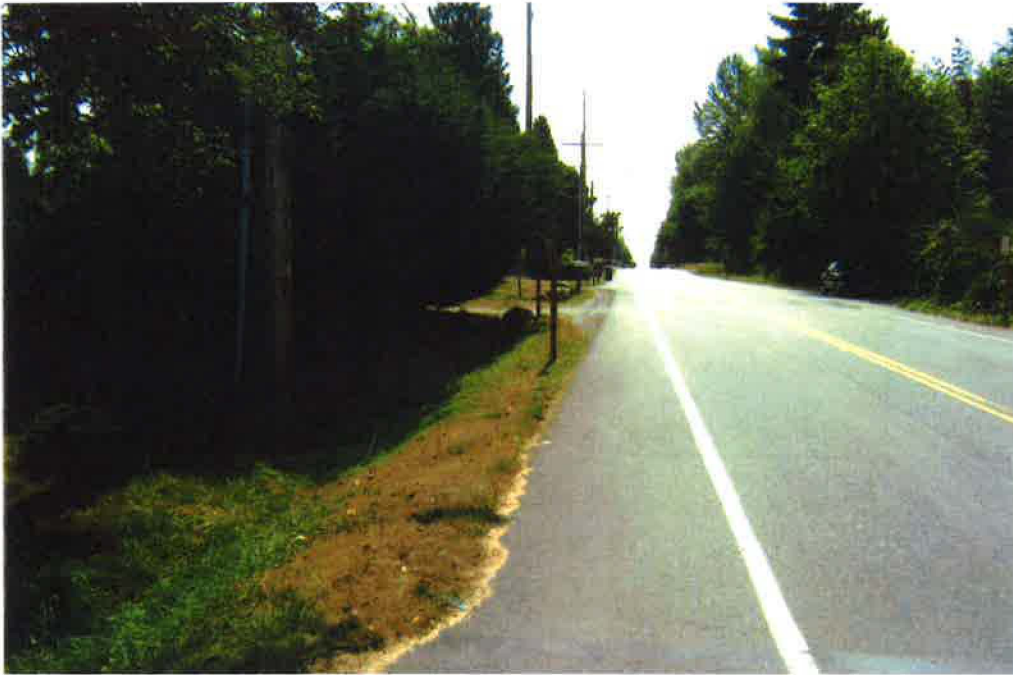
a) 24 th Ave S – S 216 th St to S 208 th St Segment before the improvements in 2014.
