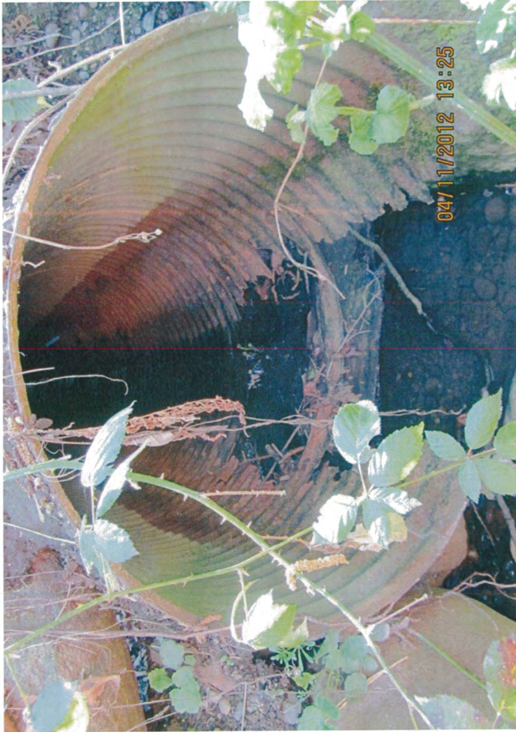
Pipe Replacement Program
