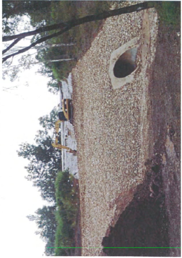
Measure 3: Rock Fill Slope
