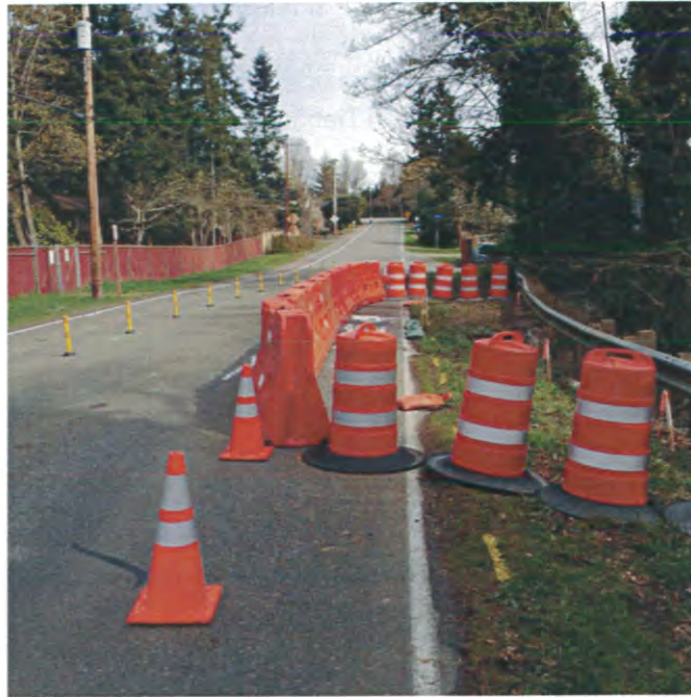
Figure 1 – Temporary Protection Measures
