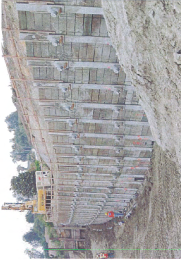
Measure 1: Soldier Pile Wall with Tieback Anchors
