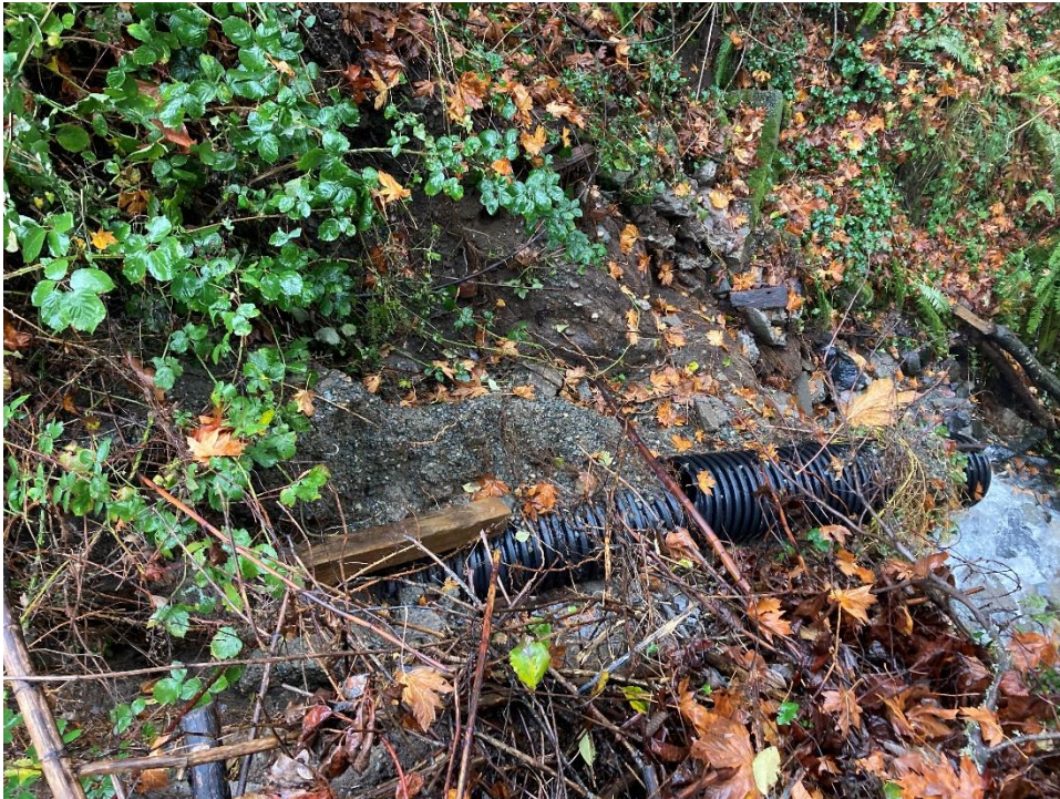
Figure 4. 256th Pl Outfall Project
