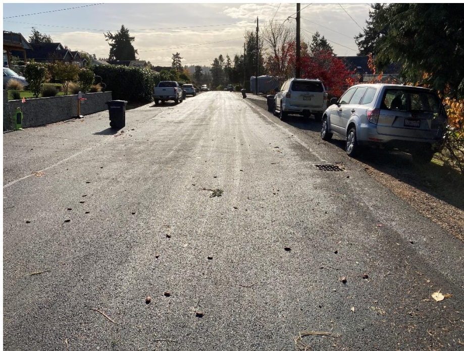
Figure 2. 8th Ave S (264th-265th) Pipe Project
