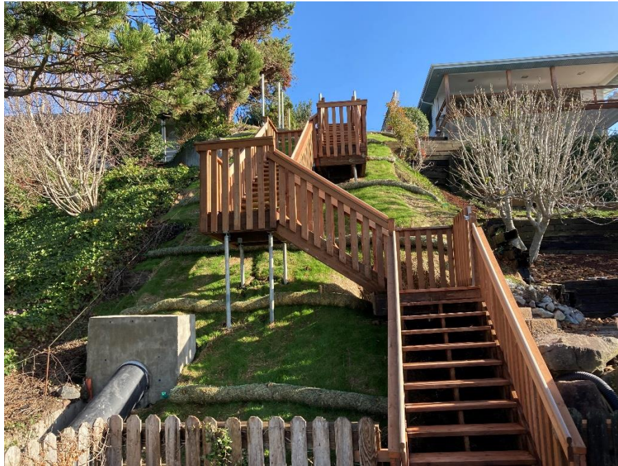
Figure 1. 239th Outfall Replacement Project
