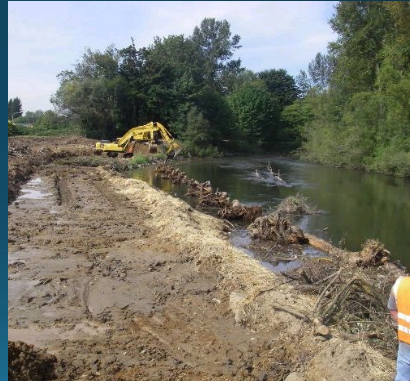
Fenster Levee Setback, Auburn
