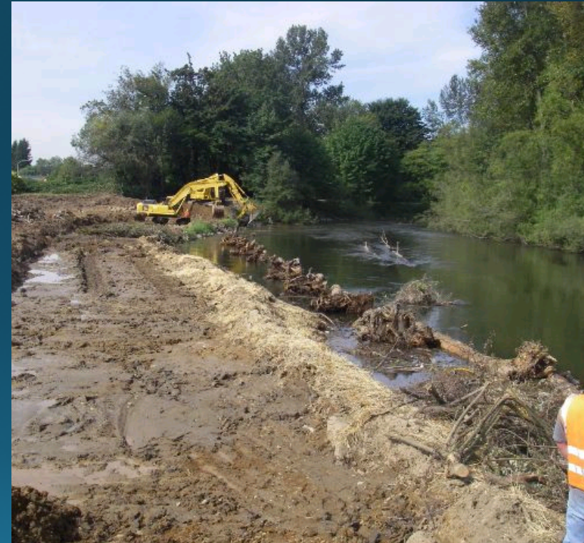
Fenster Levee Setback, Auburn
