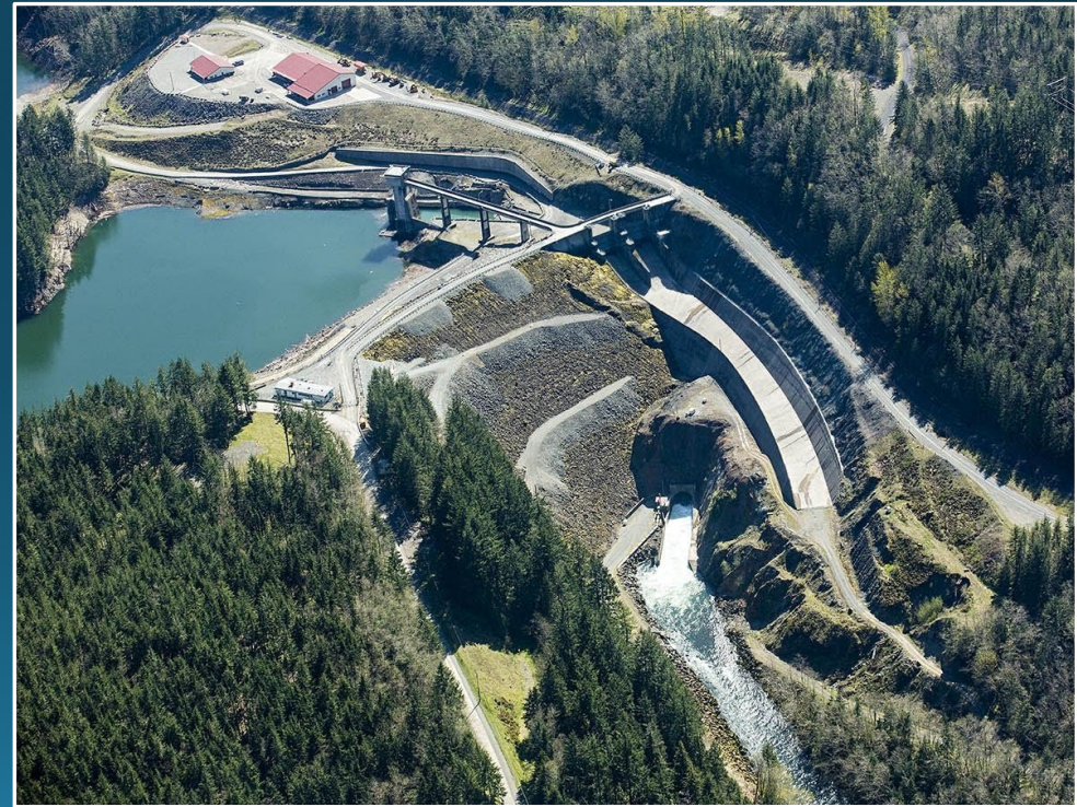
Howard Hanson Dam
