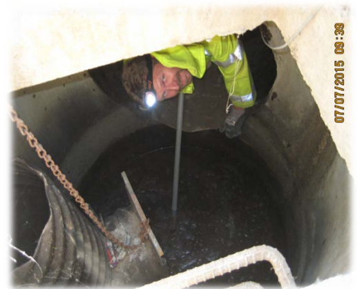
Photo 6. A SWM Public Works Maintenance Member Inspecting a Stormwater Facility
