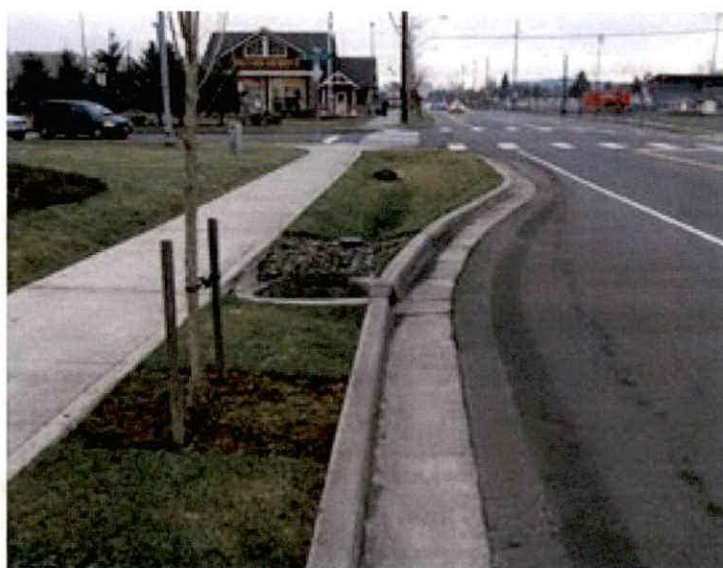
LID ELEMENTS: CURB INLETS, RAINGARDENS, CURB BULBS WITH PARKING, CENTER ISLAND LANDSCAPING
