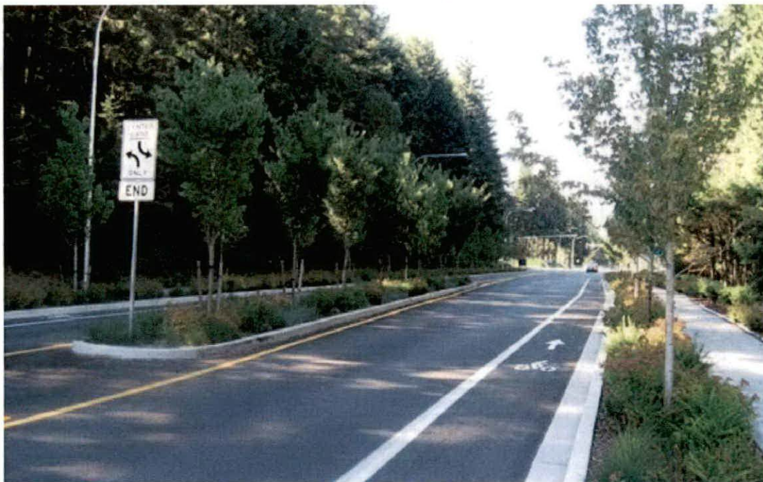
LID ELEMENTS: RAINGARDENS, PERVIOUS SIDEWALK, CURB INLETS
