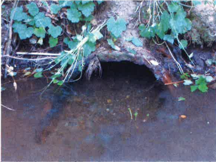
Photo 2 – Existing Culvert Outlet
