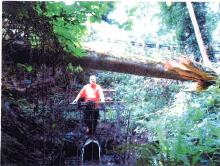
Photo 1 – Existing Culvert Entrance
