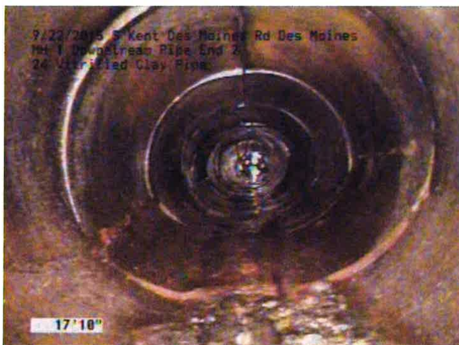
Photo 3 – Separated Joints
