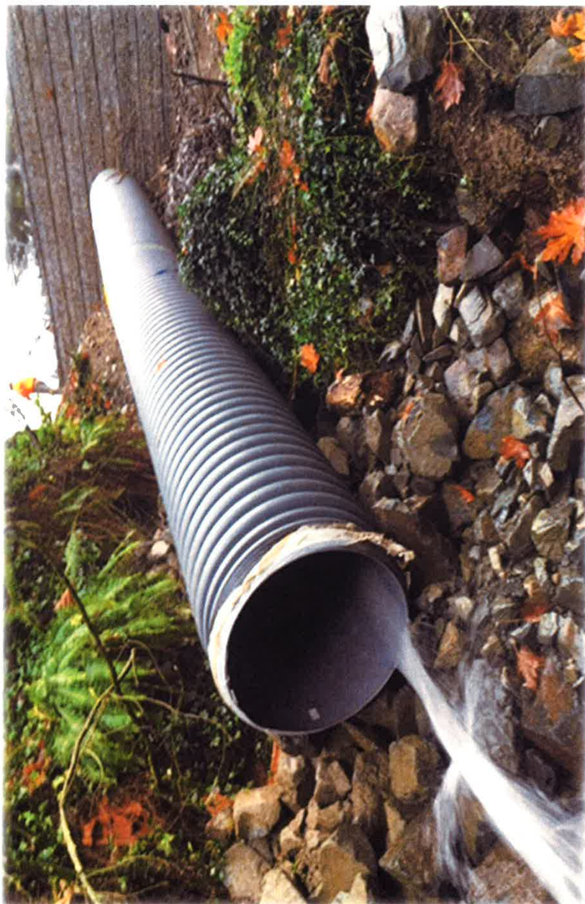
S. 251st Street Storm Outfall
