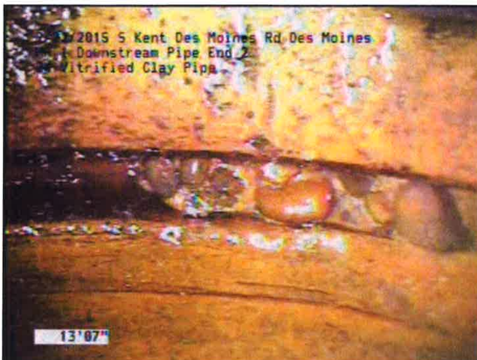
Photo 3 – Separated Joints
