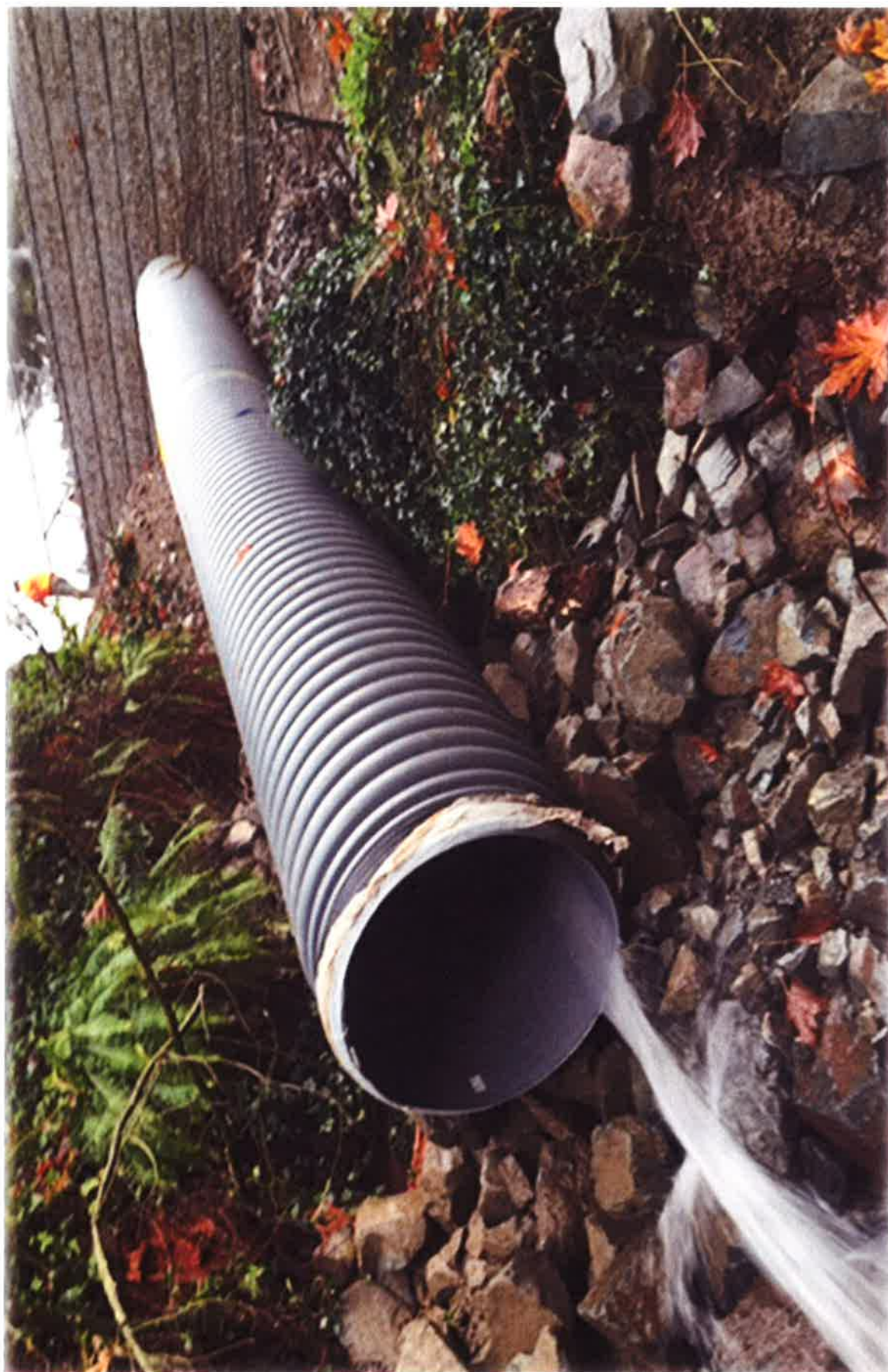
S. 251st Street Storm Outfall
