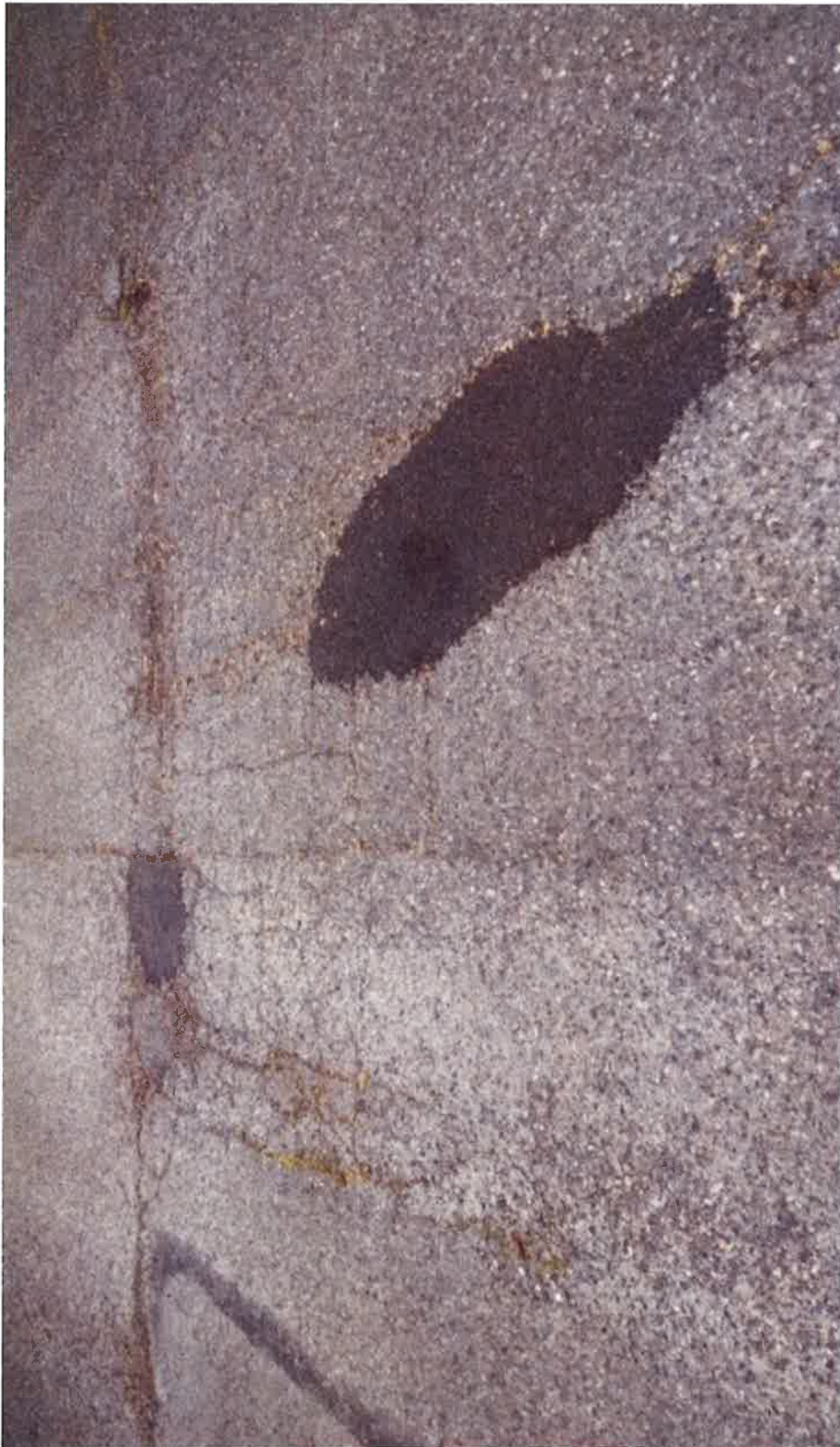
City Hall Parking Lot
