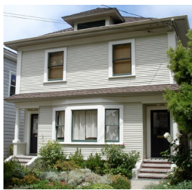
Duplex Stacked 2 units
