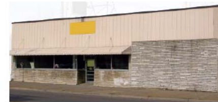
BEFORE The aluminum awning on this building is too small for the size of the building and obscures the upper portion of the windows.
