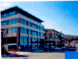
Office building almost completed
