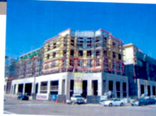
Another mixed-use building under construction
