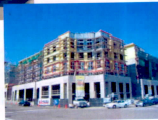
Another mixed-use building under construction
