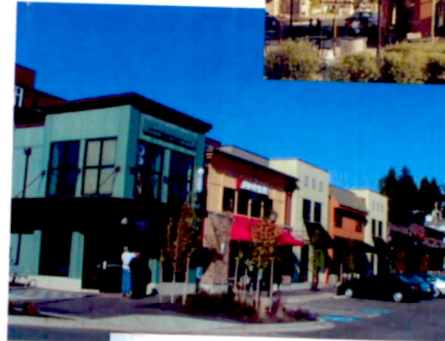
First phase of retail development
