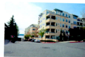
Kirkland condos with underground parking.jpg
