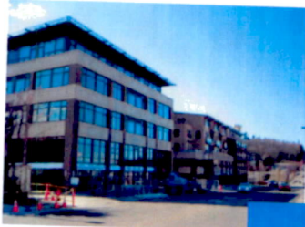
Office building almost completed
