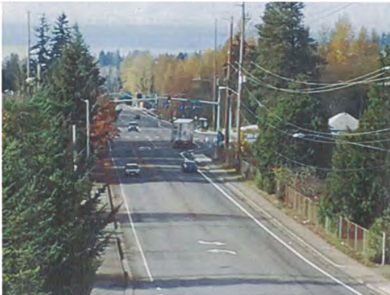
Unimproved S 216 th St looking west from SR99 (Pac Highway)
