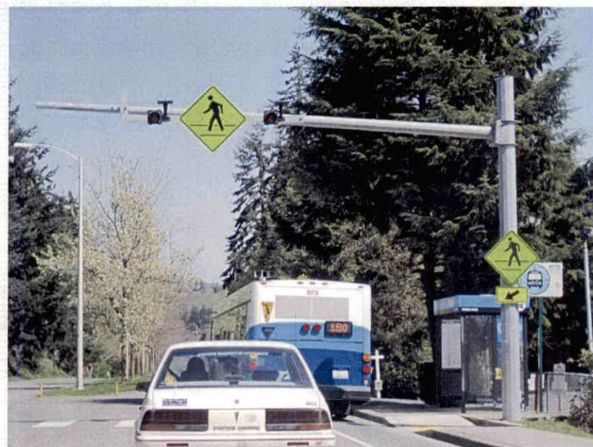
Overhead Flashing Beacon
