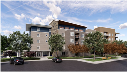
VIEW AT SOUTH MAIN ENTRANCE
